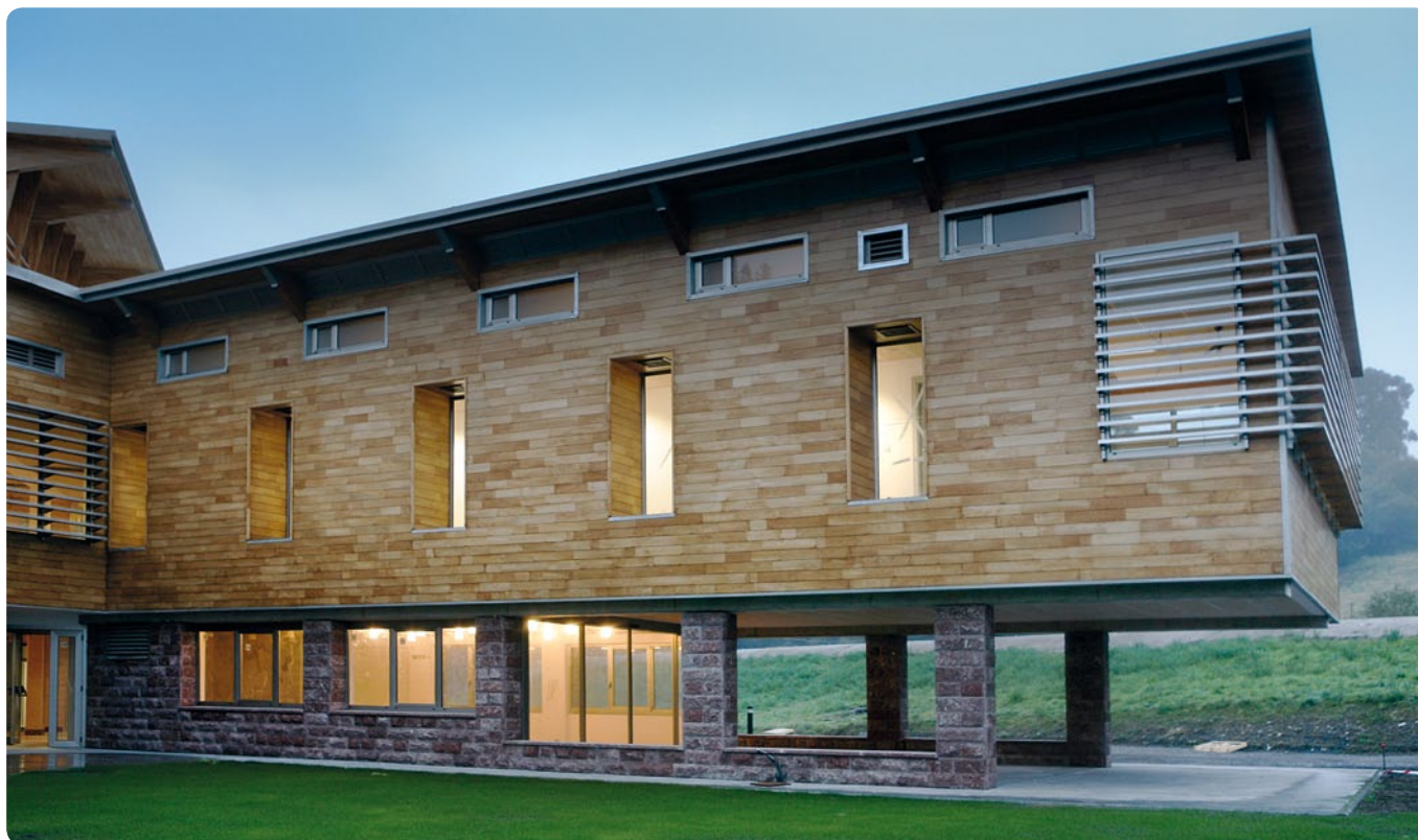
PROJECT ARFRISOL, BIOCLIMATIC OFFICES WITH SOLAR COOLING SYSTEMS.
